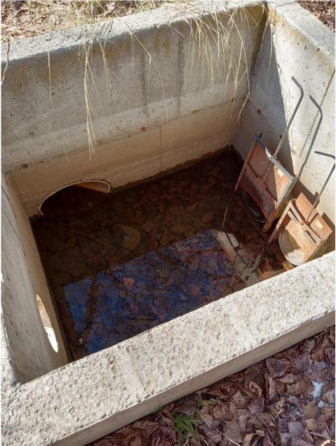
Photo A5 – Close up of Ditch 1 control valve bunker, showing typical design using baffles to direct/divert water. Note that outlet to property (left) is perched above minor trapped, standing water.
